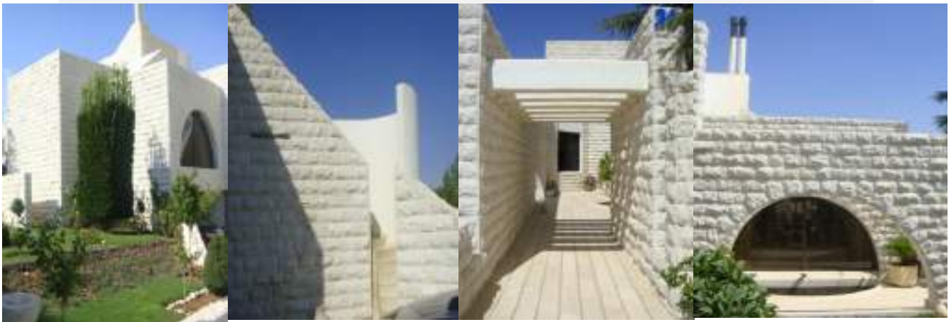
Figure (27): The general appearance of the details of the openings and stone facades in the building. Source: archnet.com.
