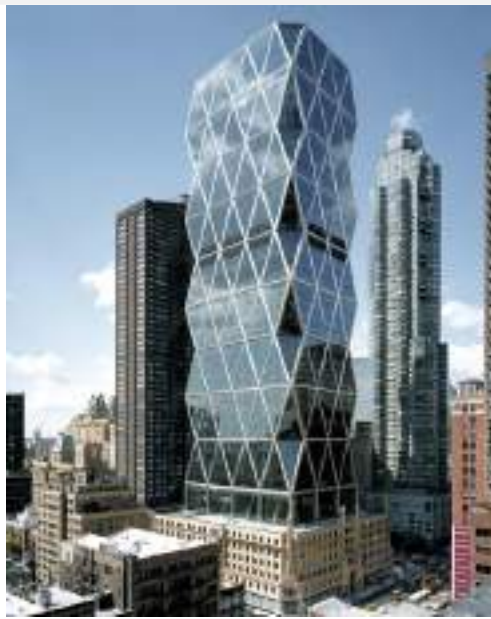
Figure (14): Hearst Tower, designed by famed architect Norman Foster (JarBot, 2022).
