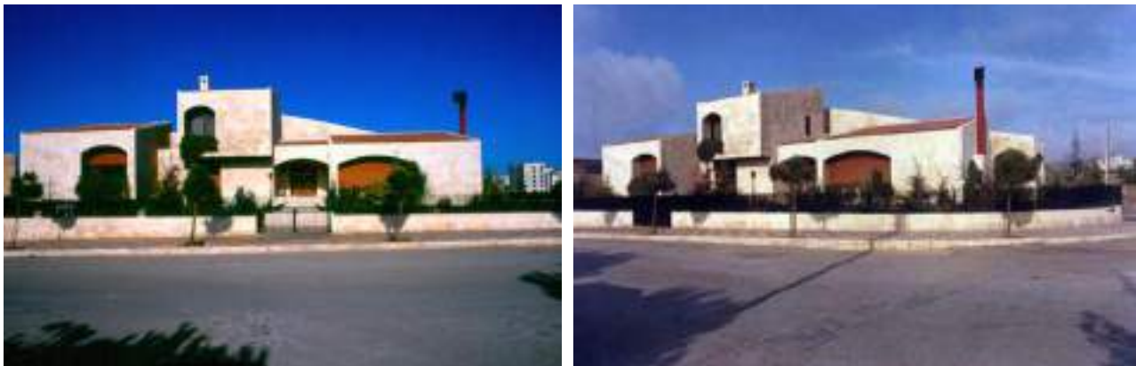
Figure (28): Villa Rizq, Jaafar Tuqan, 1980, Jordan - Amman - Jabal Amman, Total area: 870 square meters, a house on three levels: living rooms, studio, three bedrooms and a guest suite. Source: Csbe.Org
