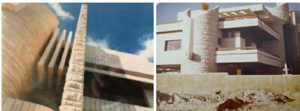
Figure (31): shows the stone facades of the building and the details of the openings in proportion to its overall shape. Source: (Arida, 2021)
